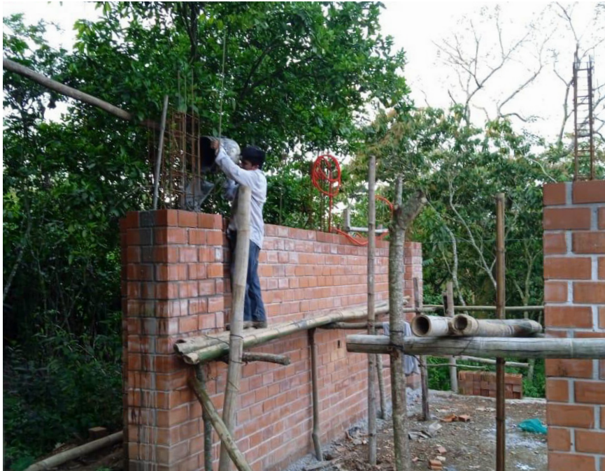
Paid labor: Casting of enclosure chain. Photo: Local crew.
