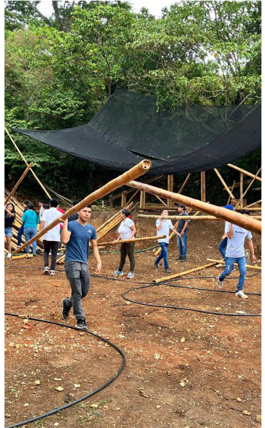
Technical training and student contribution: drying and hauling bamboo after chemical treatment. Photo: Community of students and teachers.
