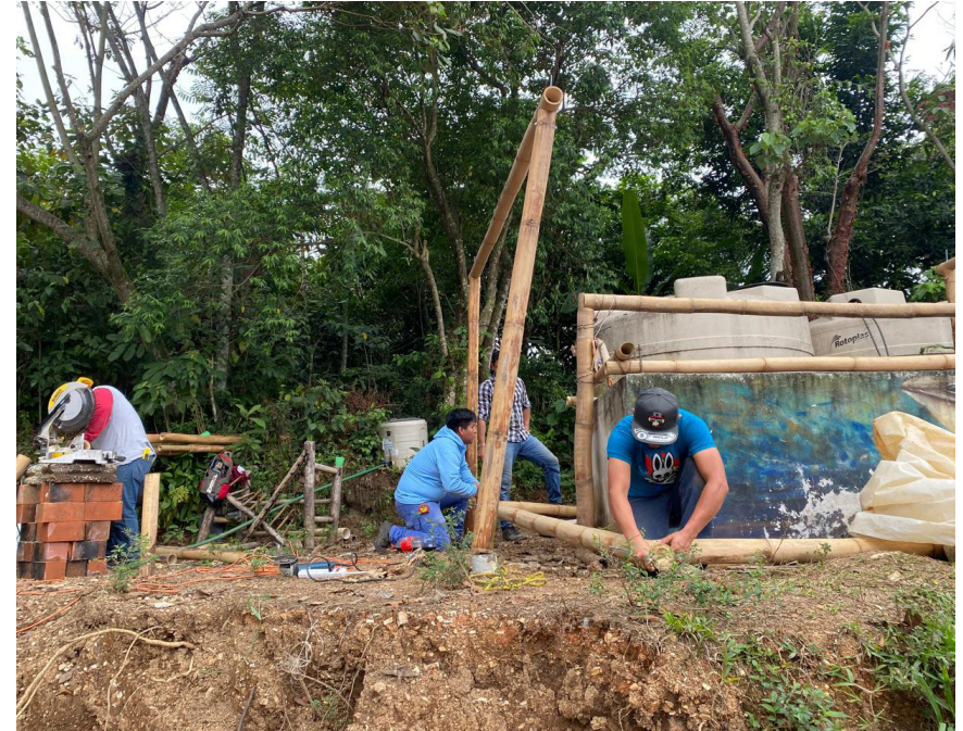
Technical training and student input: Tank roof assembly. Photo: Community of students and teachers.
