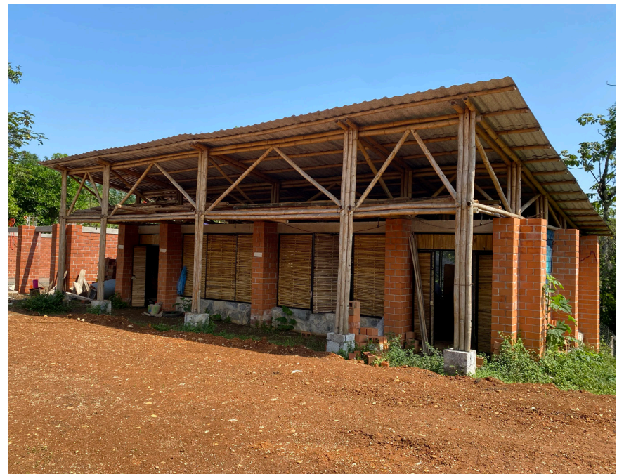
Bamboo is worn out due to exposure to the elements. Photo: Comunal
