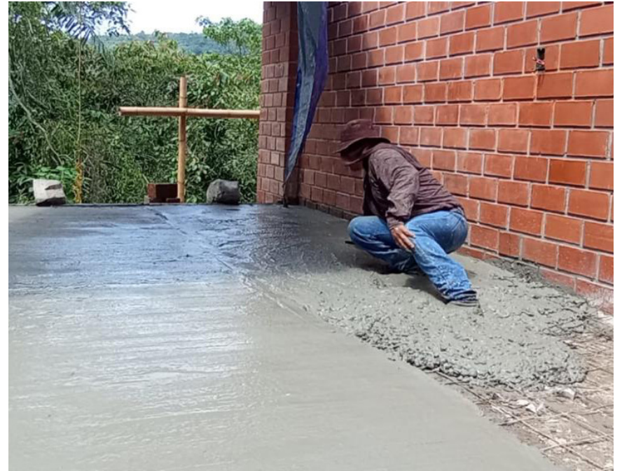
Paid labor: Slab construction. Photo: Comunal.
