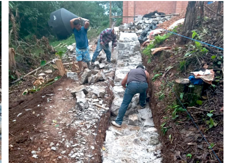
Self-employment: Construction of stone foundations. Photo: Local crew.
