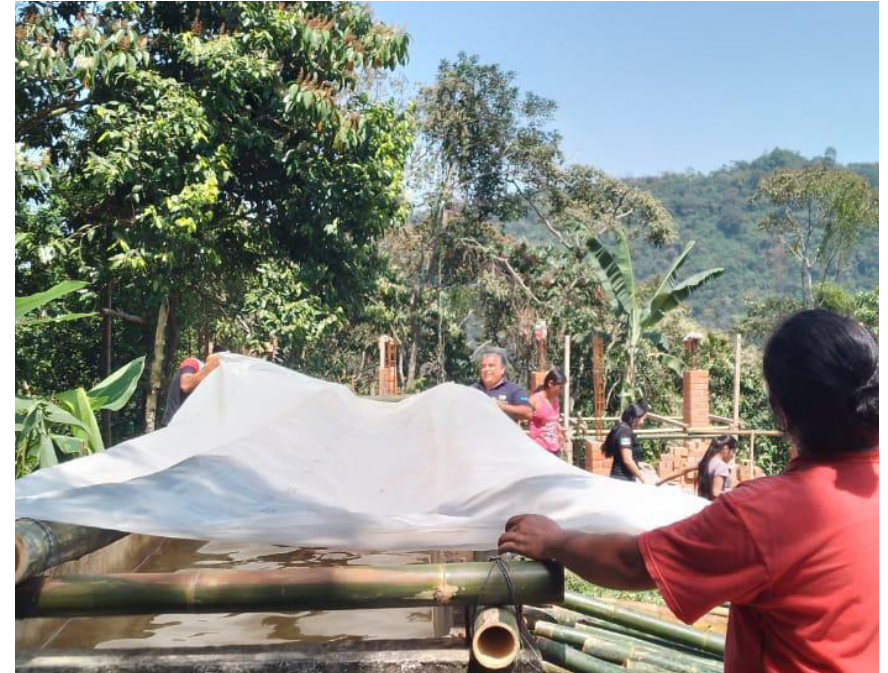
Student contribution: tank capping to avoid chemical impurification. Photo: Community of students and teachers.
