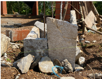
Paid labor: Construction of pedestals with flagstone. Photo: Local crew.
