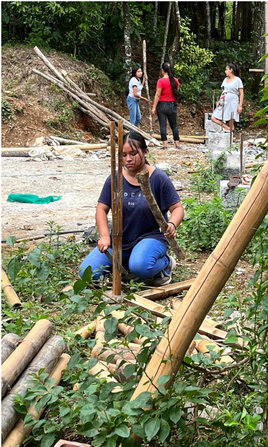
Technical training and student contribution: cutting bamboo with machete for window weaving. Photo: Community of students and teachers.
