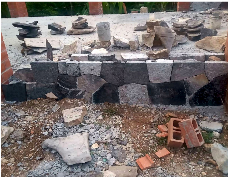
Paid labor: Construction of baseboards with flagstone. Photo: Local crew.
