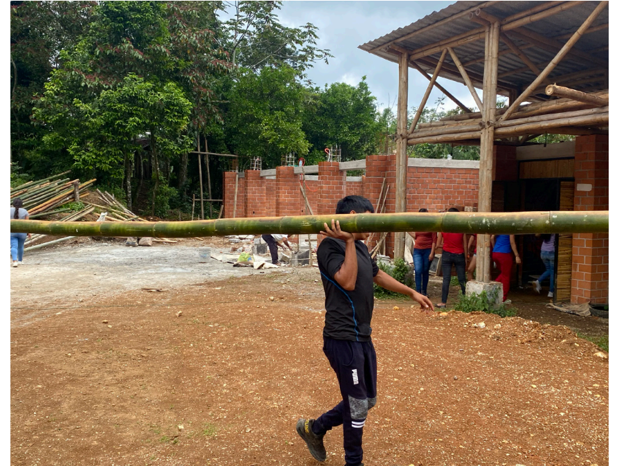
Technical training and student contribution: drying and hauling bamboo after chemical treatment. Photo: Community of students and teachers.
