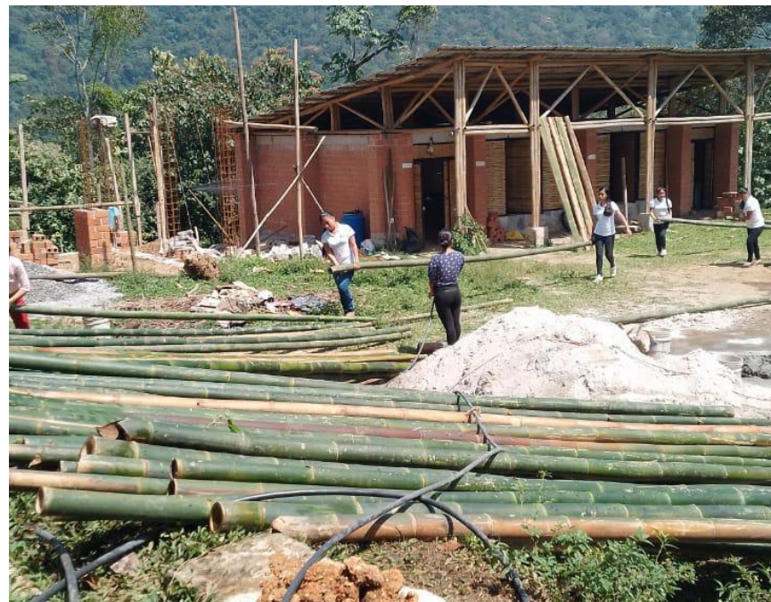
Technical training and student contribution: drying and hauling bamboo after chemical treatment. Photo: Community of students and teachers.
