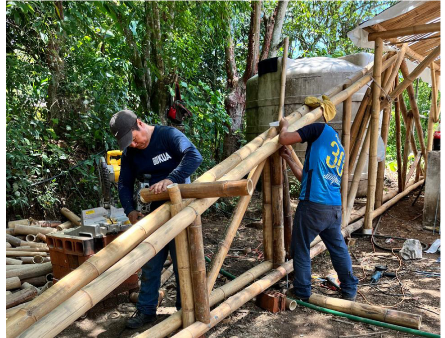
Assembly of trusses for classroom 3. Photo: Community of students and teachers
