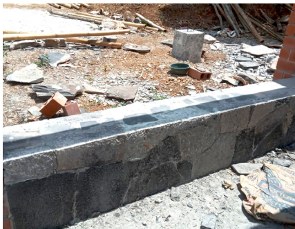
Paid labor: Construction of pedestals with flagstone. Photo: Local crew.
