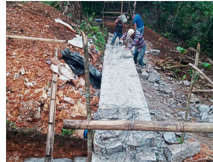
Self-employment: Construction of stone foundations. Photo: Local crew.
