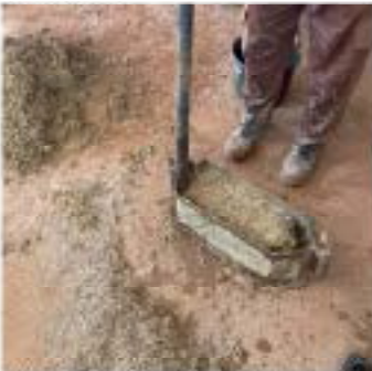
Step 5: Compacting the mix inside a metallic mold.
