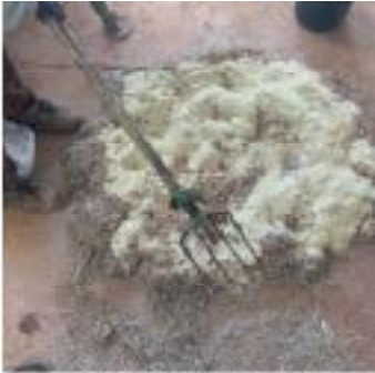
Step 3: Mixing the crushed typha with the dry clay.
