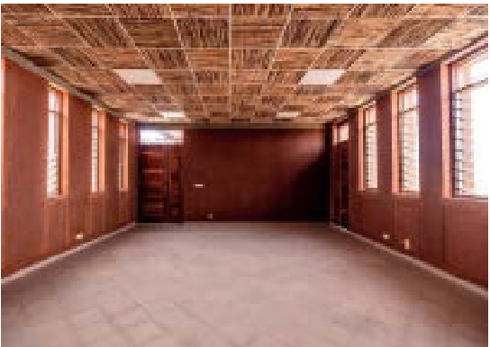
Diamniadio eco-pavilion interior with typha ceiling.
