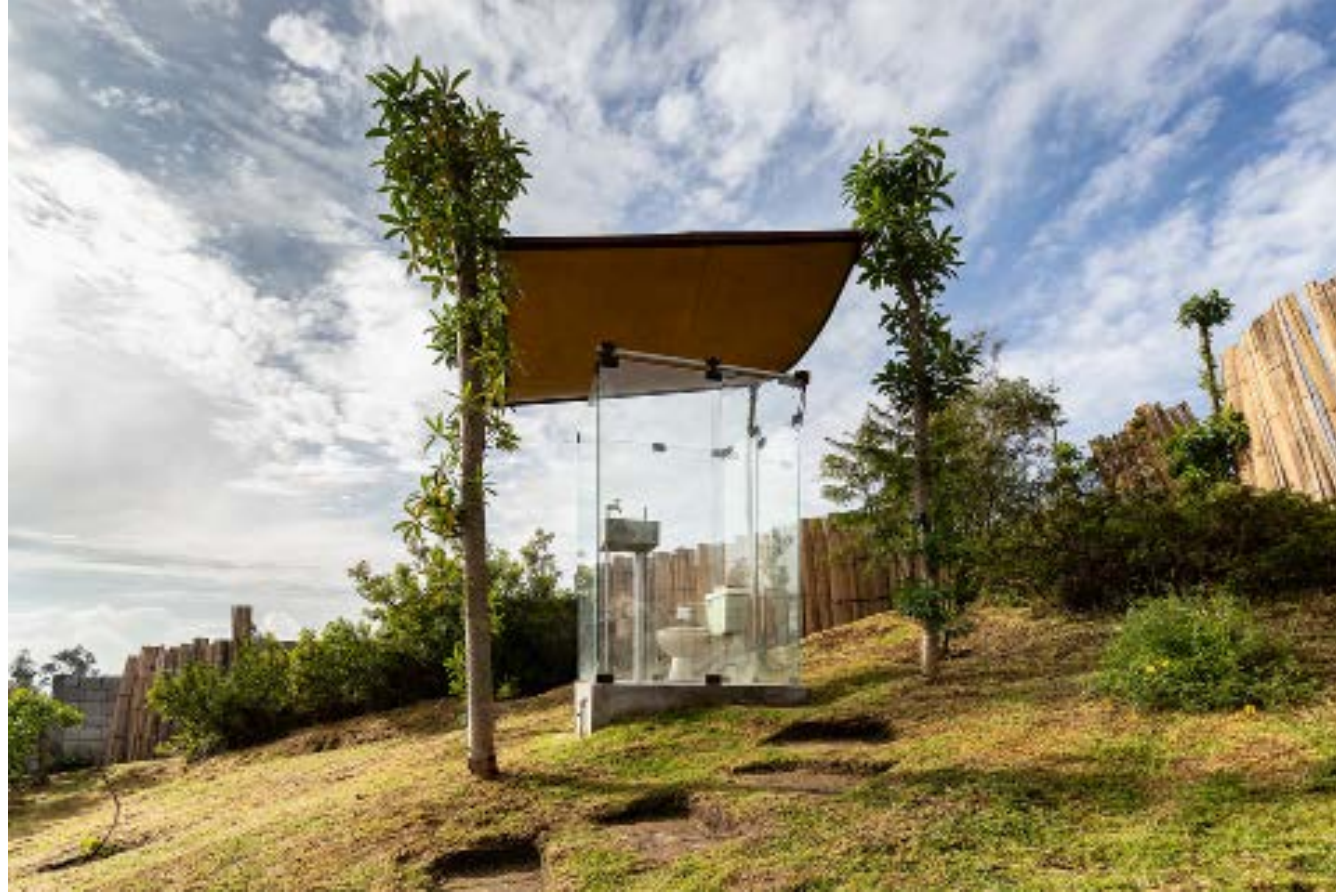
The columns of Garden House are constructed using live trees, employing a vernacular technique from the Andes region. This technique is well known for its use in building live fences. Photograph by JAG Studio
